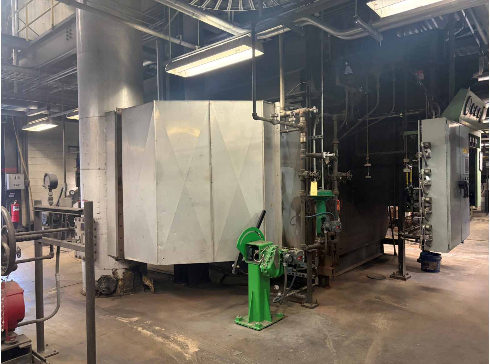
WEST SIDE WALL LOOKING NORTH EAST TOWARDS STACK AND FLUE GAS DUCT
