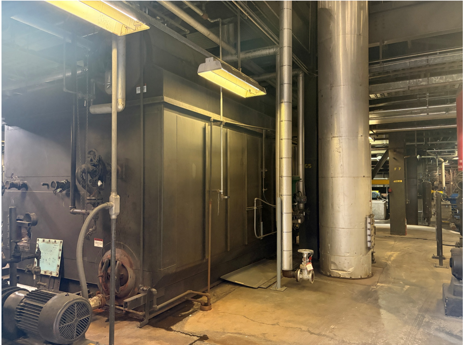
WEST SIDE WALL LOOKING SOUTH EAST
